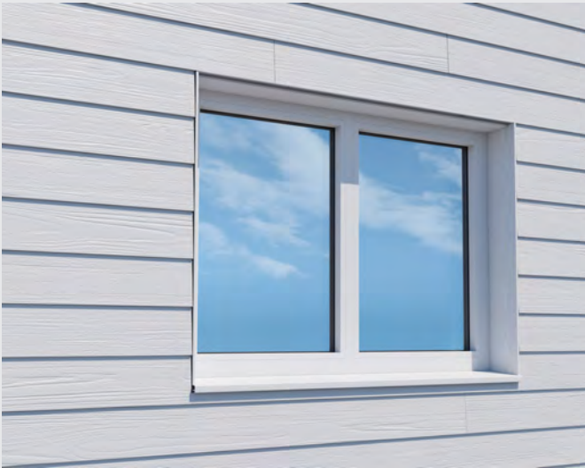
Window Detail with Hardie® Plank weatherboard on edge
