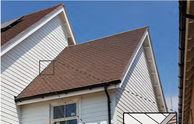
Maintain a min. 50 mm clearance between Hardie® Plank weatherboard and a hard surface eg. roofs and concrete paths, steps and driveways.
