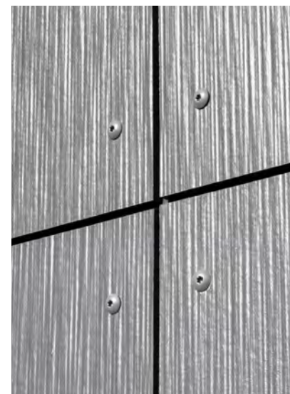
Hardie™ Panel Screw Fixing
