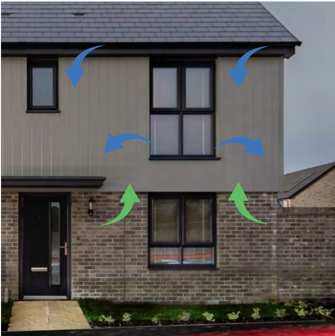
→ Green: Air inlets → Blue: Air Outlets
